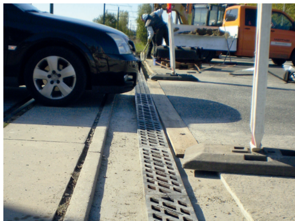
HYDROblock, Project: Spoorwegovergang, Frankfurt/Oder
